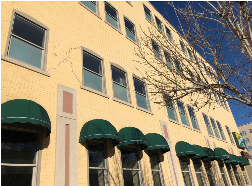
Systematic diagonal (shear) cracks appear between window groups.
