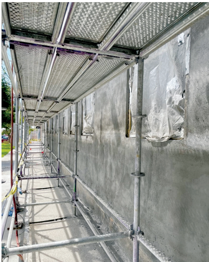
The finished FRCM application is shown after several layers of FRCM were applied and allowed to cure.
