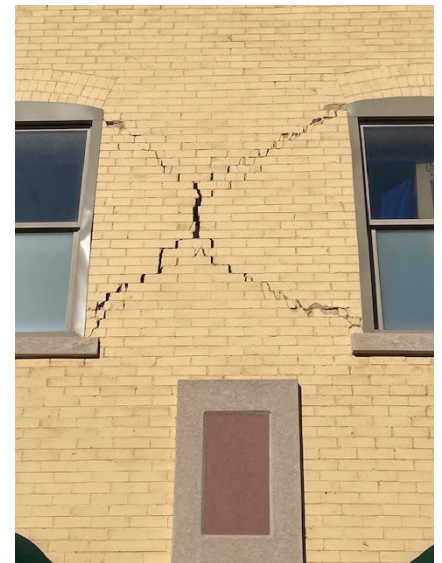
Systematic diagonal (shear) cracks appear between window groups.
