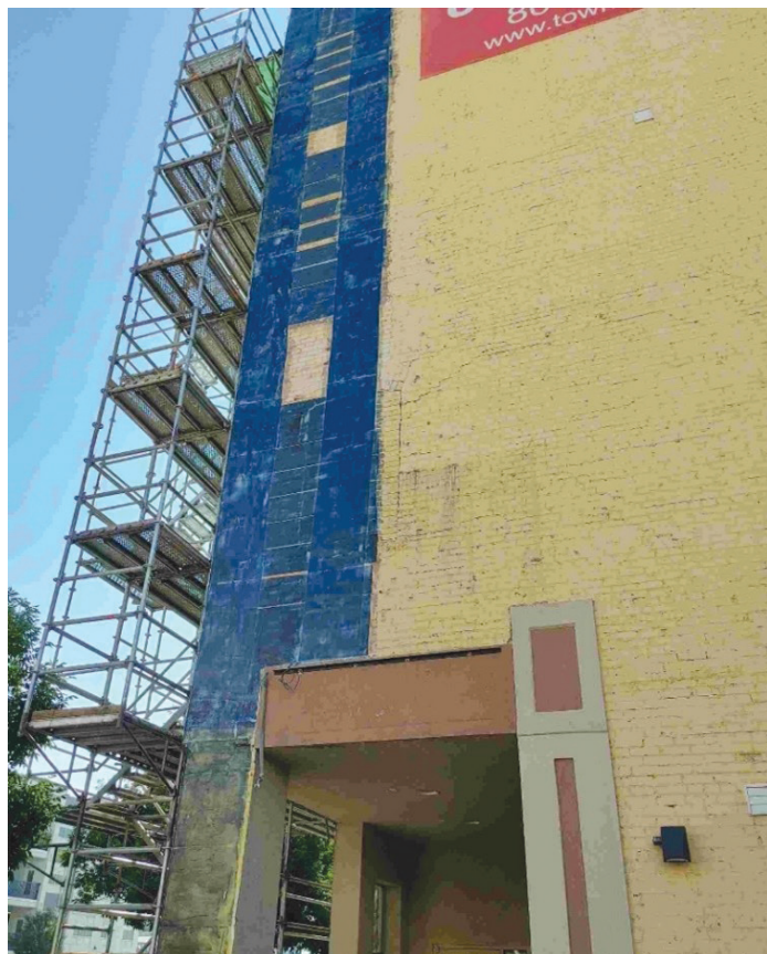
Final FRP application (dark blue) is installed in strips on the URM wall.
